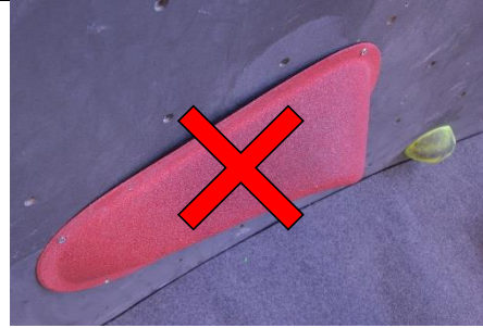
Picture 17 improper volume attachment at concave wall
