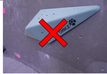
Picture 4 improper attachment at concave wall
